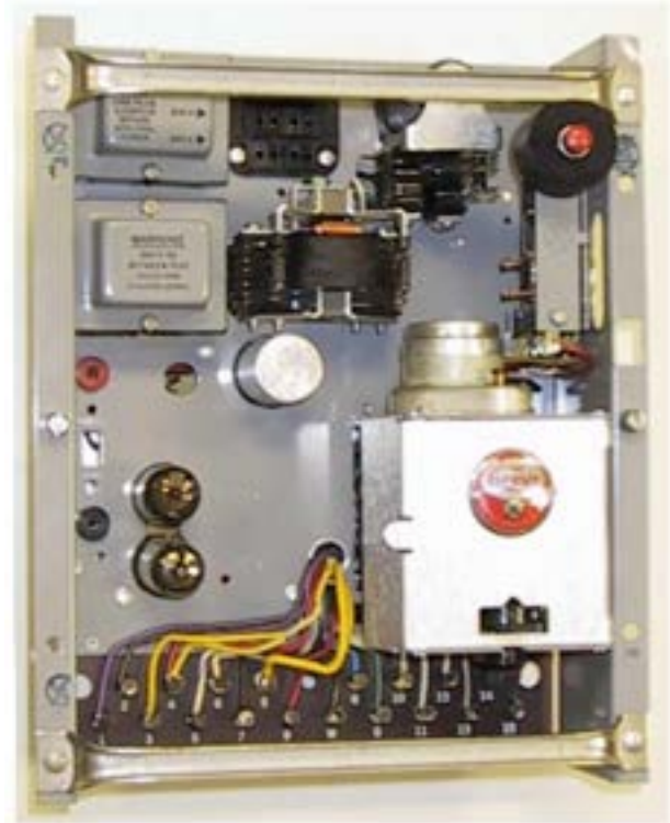
Fig. 1 Fireye P-Series control. Model: 26RJ8
