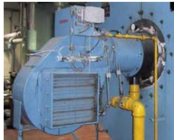
Fig. 4 Forced draft burner.
