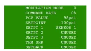
The current modulation rate is also shown here, in percent from 0% to 100%. The current PCV (process control variable) is also shown, which is the controlling sensor that the PID firing rate is based upon. The current setpoint is also shown, as well as the sensor assignments for setpoints 1, 2, 3, thermal shock and setback.
