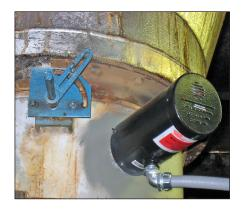
The package supplied included a PPC4000 controller, NXD410 display, 3 FX servos and NXCESO2 Oxygen probe.
