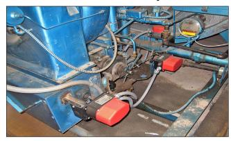
The system was installed on a 350 HP Superior Scotch Marine boiler with an IC burner. The Industrial Combustion burner fires natural gas and #2 oil.
