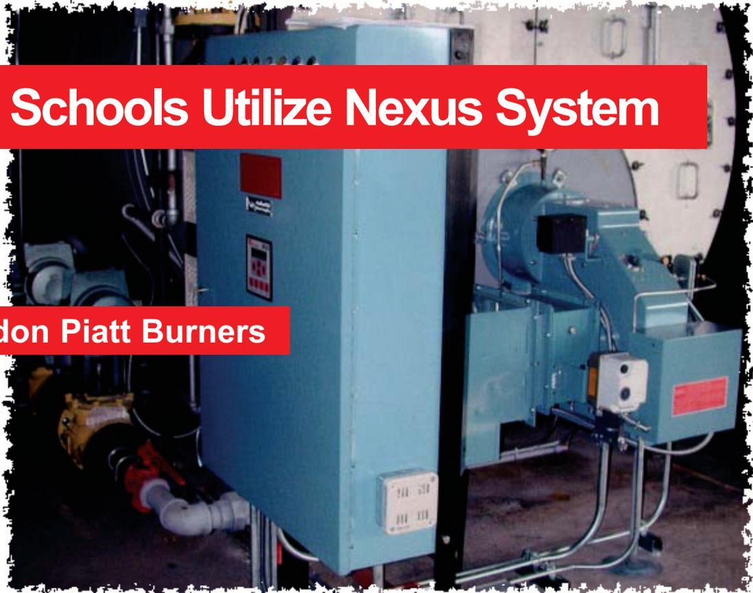
Four new Gordon Piatt gas burners were fitted at two schools in Detroit, MI to update their existing firing systems. Each of the burners was supplied pre-fitted the Fireye Nexus control system. The Nexus system offers fully integrated control, providing burner management in one low cost package.
