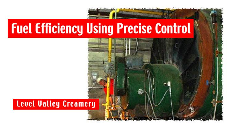
A Nexus burner control system was fitted to the Johnston boiler/burner combination at the Level Valley Creamery in Nashville Tennessee. The 900HP boiler was original-
