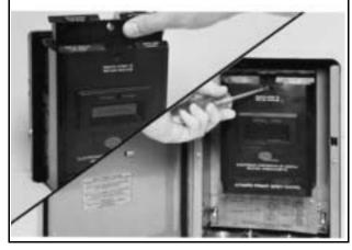
**5.** Replace the Firetron cell in the scanner with the #4-263 Firetron cell.
