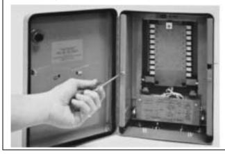
**5.** Replace the #4-128 Firetron cell in the scanner with the #4-263 Firetron cell. Attach the label supplied with the #4-263 Firetron cell, to the scanner body.
