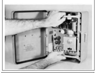
**4.** Assemble the control and modules and install the unit into Moderization Adapter. Tighten the chassis retainer
