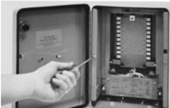
5. Assemble the control and module and install the unit into the Modernization Adapter. Tighten the chassis retainer.
