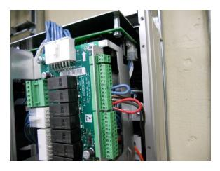
Install Jumper on terminals 1& 2.
