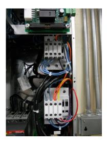
Install M2 & M3 contacts and wire to FSG or Integrated Control Contact shown. GE P/N BCLF10 (N.O.)
