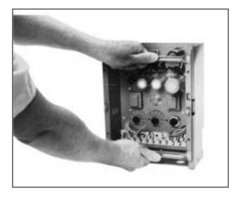
4 Insert modules in Control chassis and install into Modernization Adapter. Tighten the chassis mounting screw.
